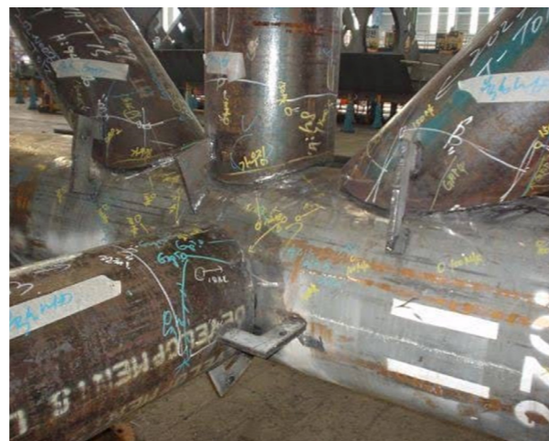
DTDK joint showing the complexity of welding offshore nodes with limited accessibility and a variety of welding positions.
